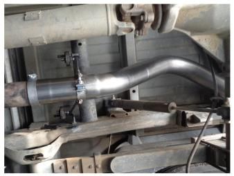
**Step 4.** Next, loosely slip the Hanger Clamp Assembly over the Over Axle Pipe. Loosely secure using the supplied clamps. Engage the welded hangers of the Hanger Clamp Assembly to the rubber insulators.
