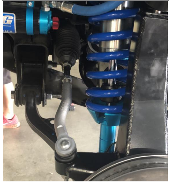
Figure 46d: Tie Rod End Installed (Driver's Side Shown)
